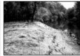
Restoration included removing Japanese knotweed regrading the bank, installing fiber matting and biologs, and replanting with native grasses, shrubs and trees.
