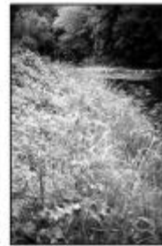
Restoration included removing Japanese knotweed regrading the bank, installing fiber matting and biologs, and replanting with native grasses, shrubs and trees.
