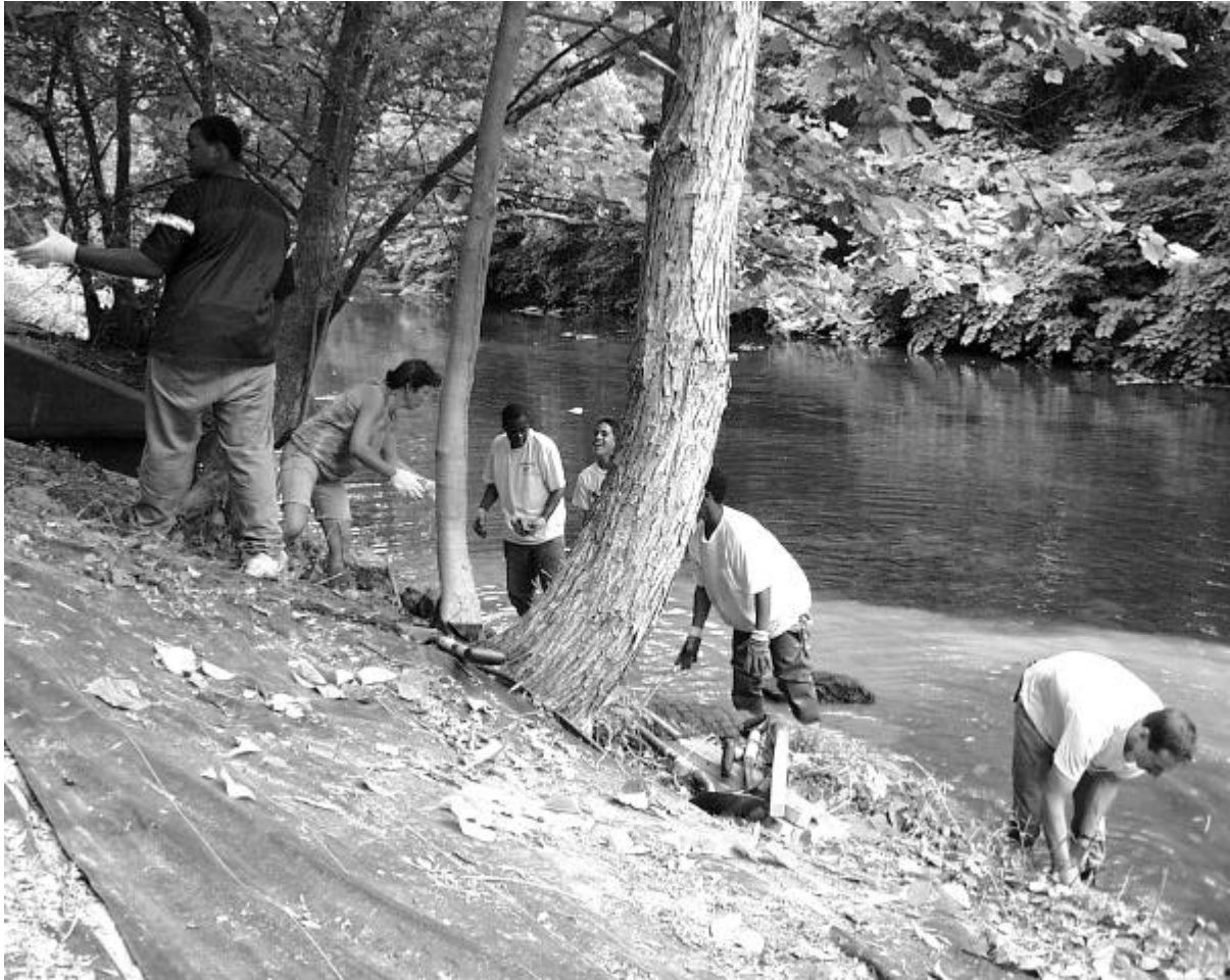
Stream bank stabilization in progress.
